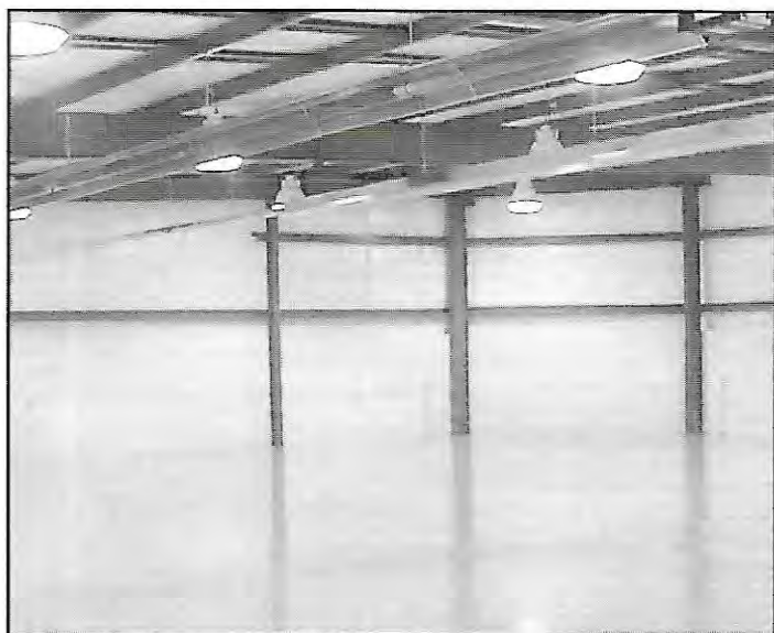
A 5,000-square-foot storage and archive building was added behind the old body shop at Templeton Hall. More renovations for Templeton are scheduled for the summer '02. Photo by Janelle Flory
