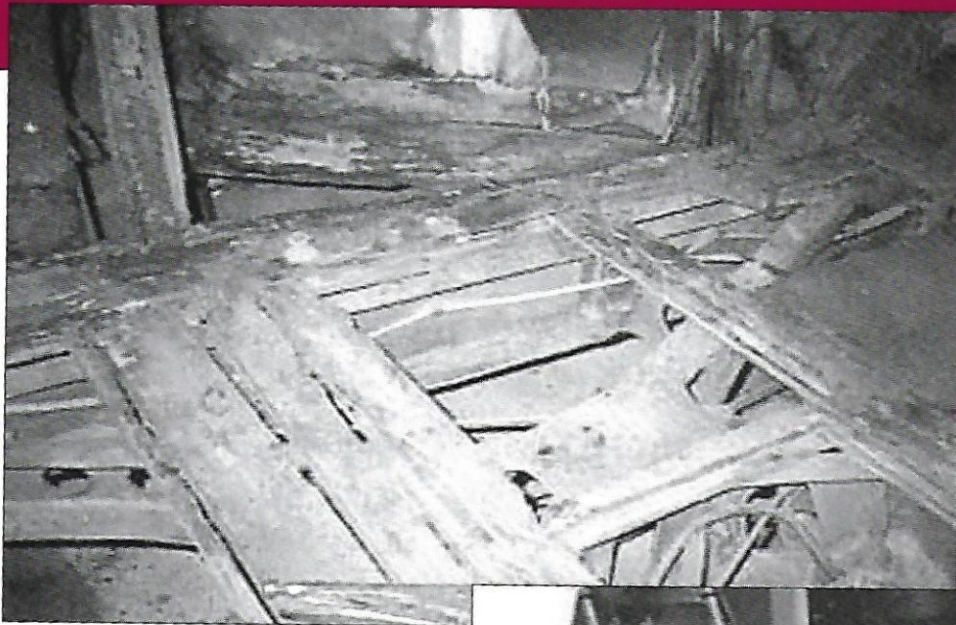
Sped along by effects of flood damage, the original wooden floorboards and frame (at left) show the deterioration of time. Mounts and his students reconstructed and installed the floorboards below.
