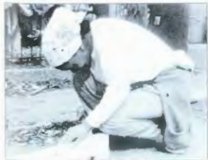
Munira Hamud-Socoro is intense about her work, lining up two boards to make the perfect right angle.
