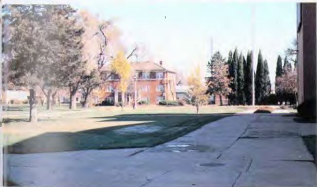
With the renovation plans came the news of the demolition of one of the most popular halls on campus, Arnold.
