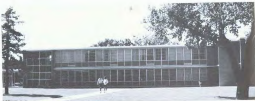
MOHLER HALL...Rating of philosophers, historians, and bookkeepers takes place upstairs with routine administrative business being handled on first floor.
