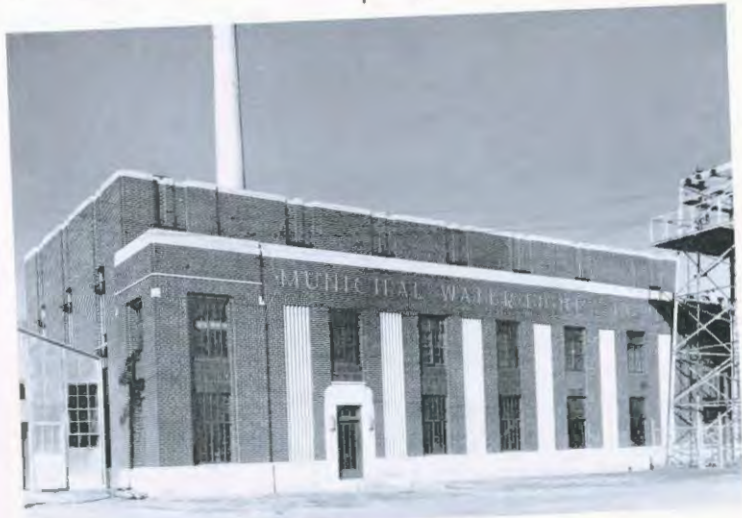
Exterior View of McPherson's Municipal Electric Generating Station
