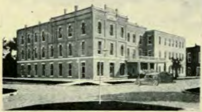
County Hospital—Carnegie Library—Junior High School—Y. M. C. A.—Street Scene—Hotel Building.
