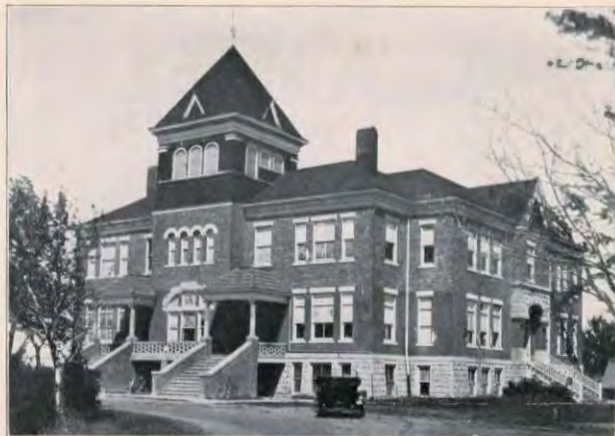
SHARP ADMINISTRATION BUILDING.
