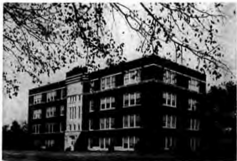
HARNLY HALL —a modern classroom building with well equipped laboratories. Chemistry, biology, physics, math, the social sciences, and music are taught here. The college museum, with the world's largest synthetic diamond, is on fourth floor.
