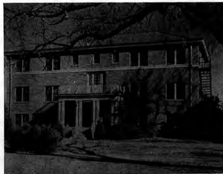
KLINE HALL —a combination apartment building for college married couples and a girls' dormitory.
