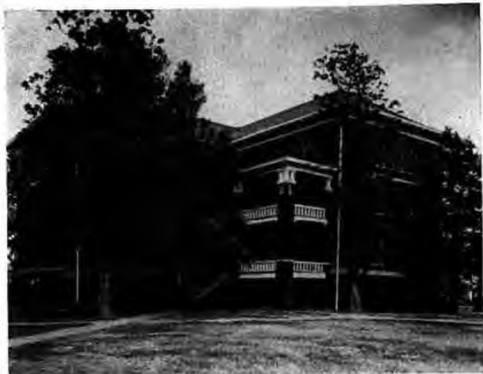
ARNOLD HALL—a large well equipped dormitory which provides for 66 men and also space for a modern cafeteria.
