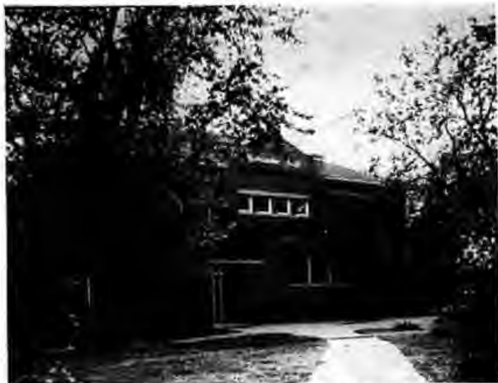
LIBRARY —One of the best equipped libraries in the midwest. Originally a gift of Andrew Carnegie it was enlarged and completely modernized in 1950.
