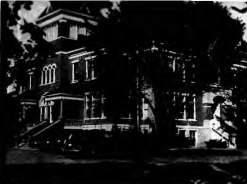
Sharp Hall - Administrative Offices
