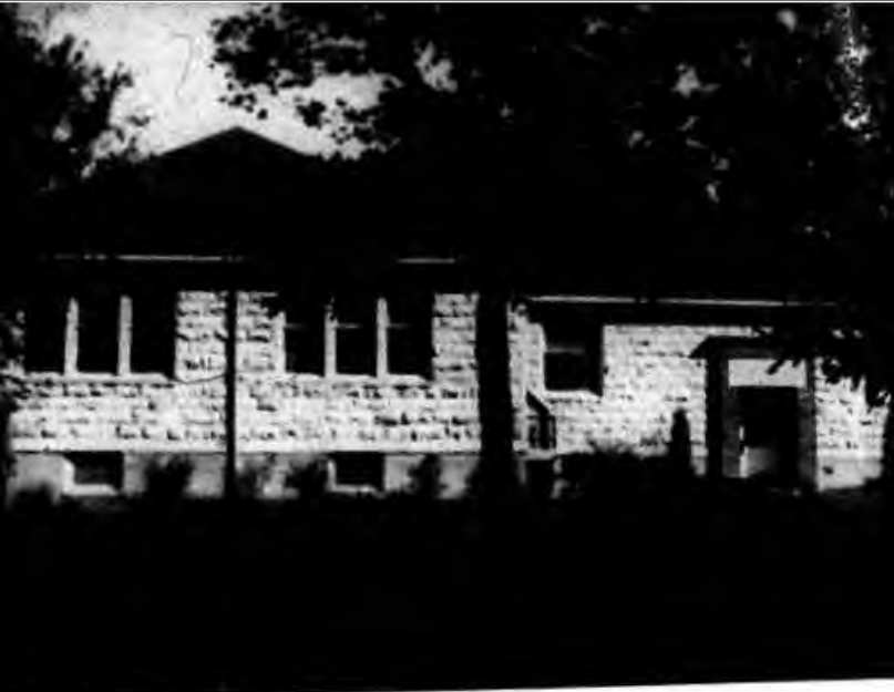
Frantz Industrial Arts Building
