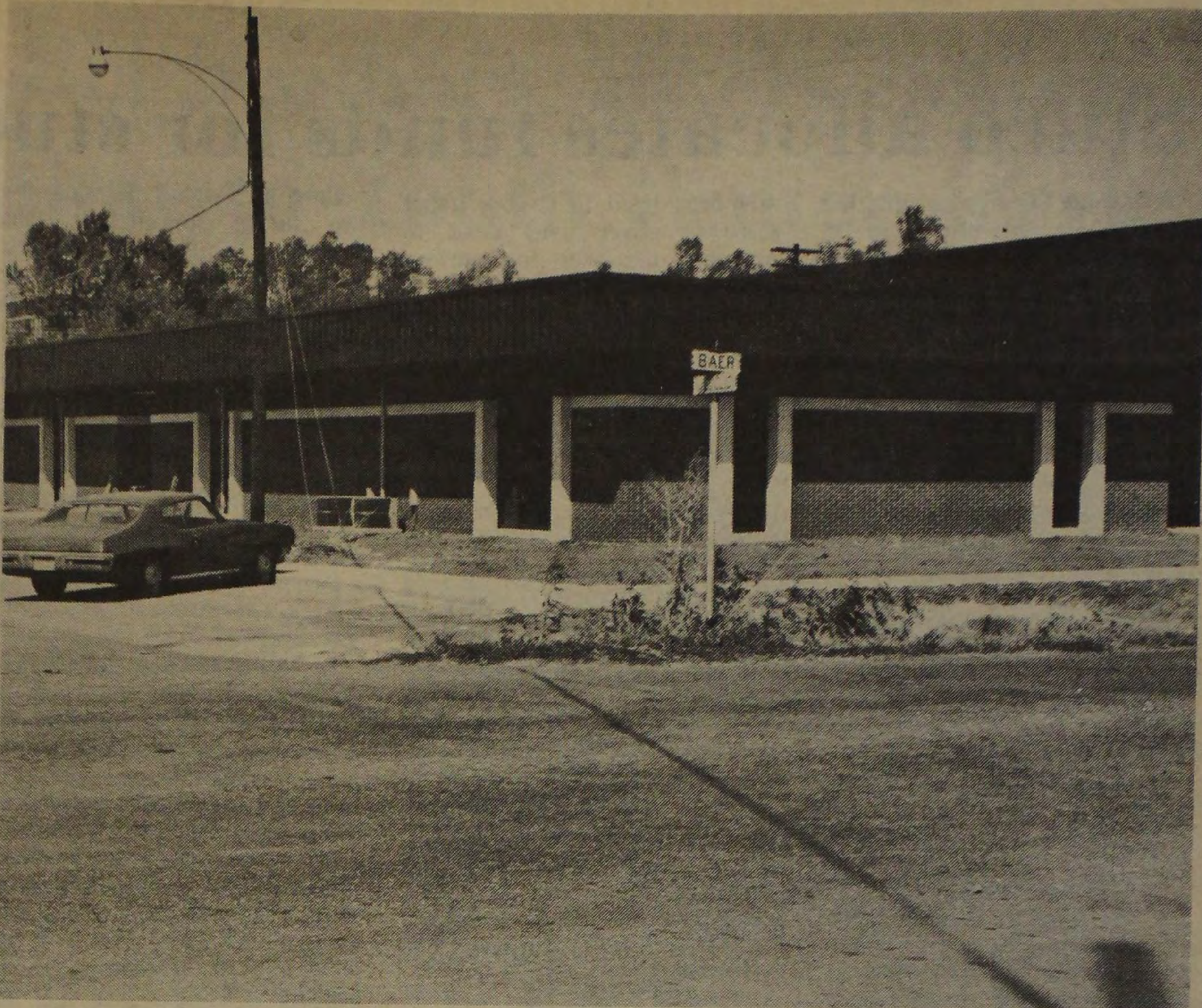
After a year of construction, the new Industrial Arts Center is ready for partial habitation. The structure will take place gradually throughout the semester. The building is located north of Metzler and Bittinger Halls. (photo by Rhodes)
