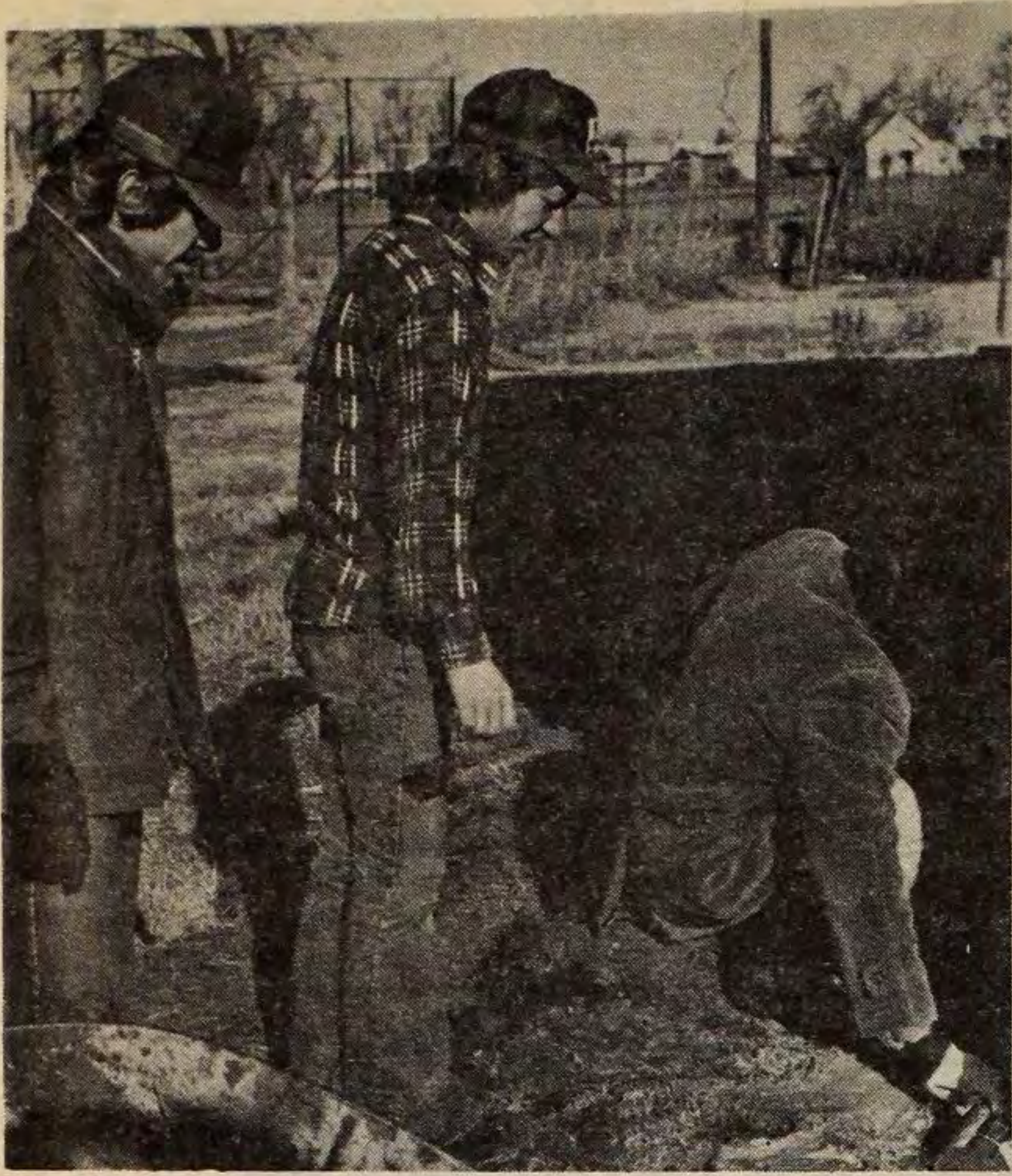
Harold Rose, Larry Brubaker and Milt Goering help with concrete foundation for Mac Shack. Johns-Manville has donated the insulation for the building.
