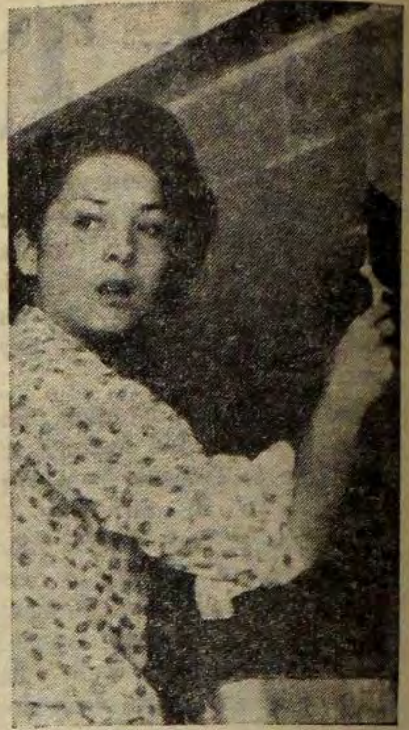
Mary Hoover gives the ceiling a coat of red paint as the WAA turned out to paint the girls locker-room.
