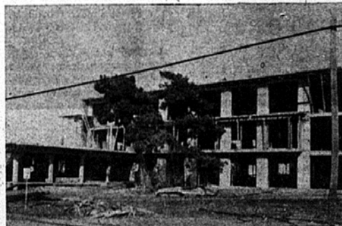
TWO GNARLED CONIFERS—add a touch of the old to the new men's residence hall being constructed east of Farnestock Hall. The dormitory is scheduled for completion before the fall semester and will house 158 men.
