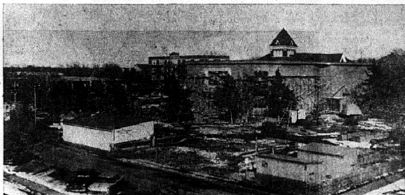
This aerial view of Brown Auditorium and Mohler Hall was taken in January just as masons had completed the brick laying of Brown Auditorium and were starting on Mohler.
