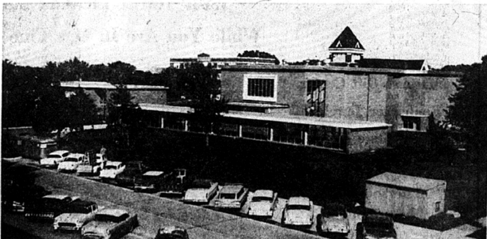
The completed buildings as they appeared on Wednesday of this week were started some twenty months ago in March, 1959 and cost over $900,000. Mohler Hall is used for administration offices and classrooms, and Brown contains the college music department along with the auditorium.
