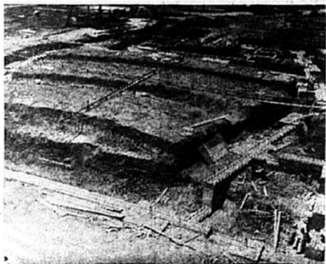
Construction work on the new Brown Auditorium was moving ahead with speed as this picture was taken in late June, 1959. Footings and walls for the auditorium were just being completed.
