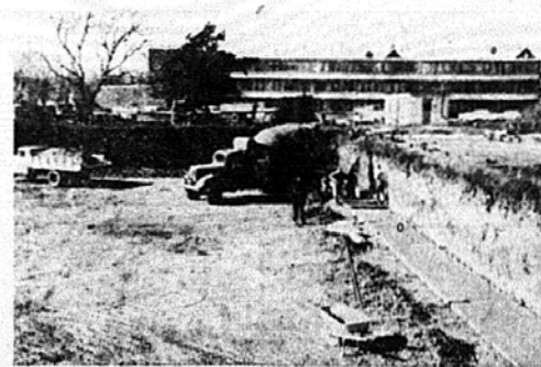
Excavation work has been completed and concrete footings are being poured for the new student union-cafeteria, on the left, and the addition to Dotzour Hall, girls dormitory. Johnson Builders, Inc., Salina, began work on the new buildings before Christmas. The excavated area for the student union will house student recreational facilities, student organizations offices, a large lounge area, a TV room and cafeteria storage area. The
