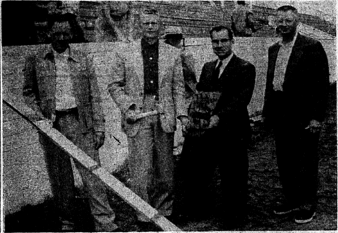
"OPERATION TEAR-DOWN" began Monday afternoon, as college officials initiated the project. Shown here is President of the College D. W. Bittering after he pulled the first slat from the condemned stadium. Construction superintendent Harold Johnson, Coach Sid Smith and John Casebeer look on. The stadium was completely torn down Wednesday evening.
