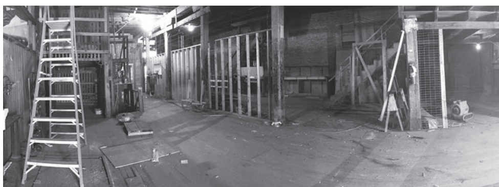
Looking in from the back door of the building.
